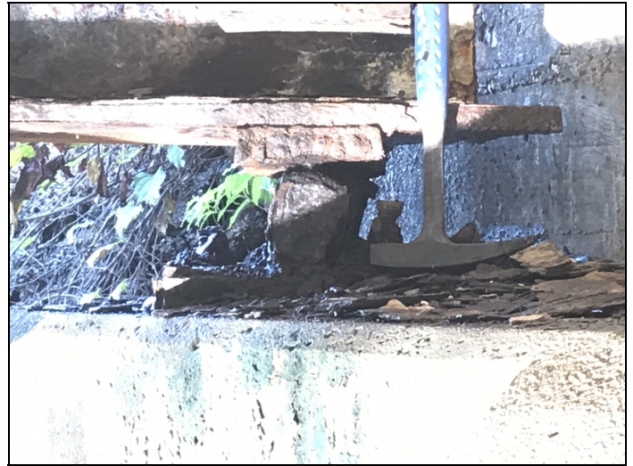
Bent 2 girder 1 bearing leaning 2019
